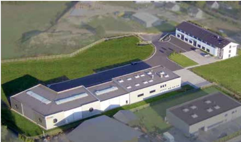
Plant Nümbrecht - Germany
